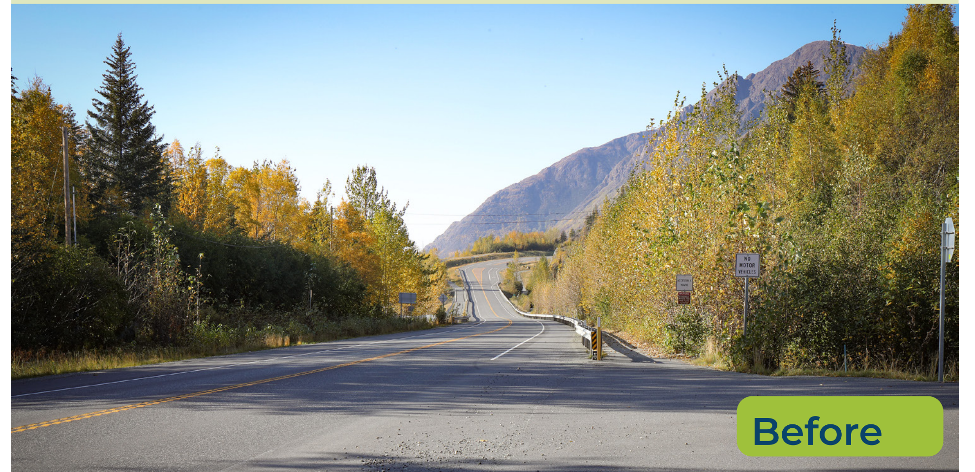
Bird Creek Looking North
